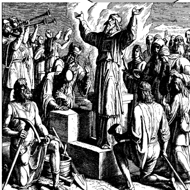
Rebuilding the temple. 676
